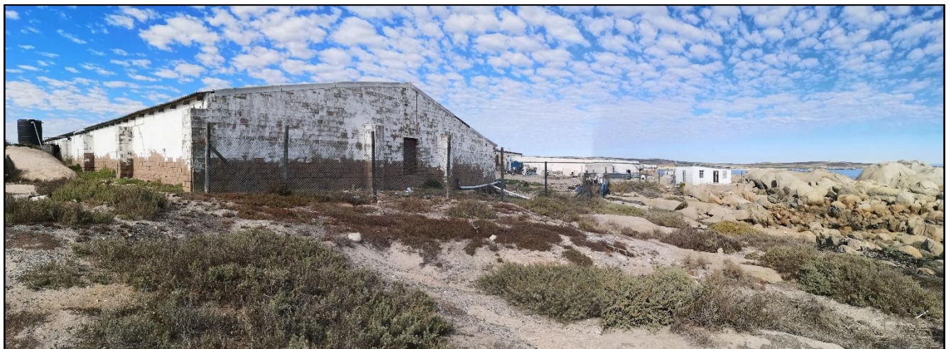
Figure 4: Existing buildings from the northwest
