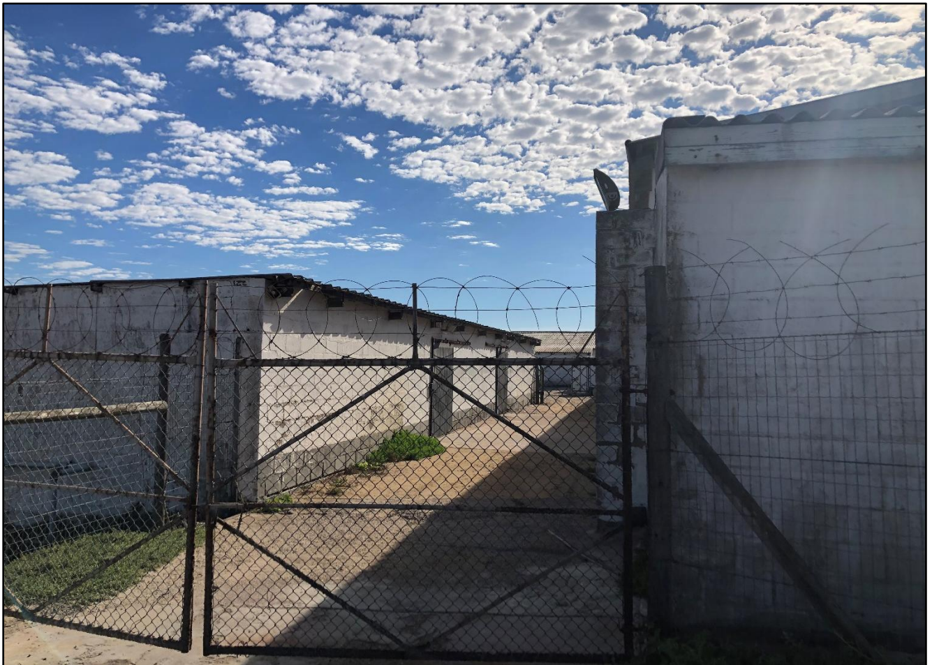
Figure 2: Existing buildings from the south
