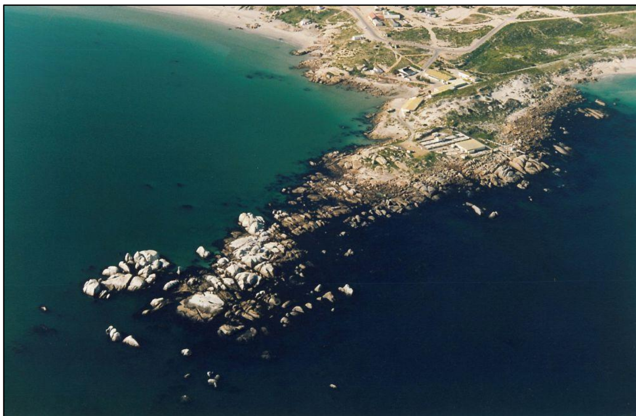
Buildings and structures on the project site with the crayfish holding building in the right foreground (circa 1980)
